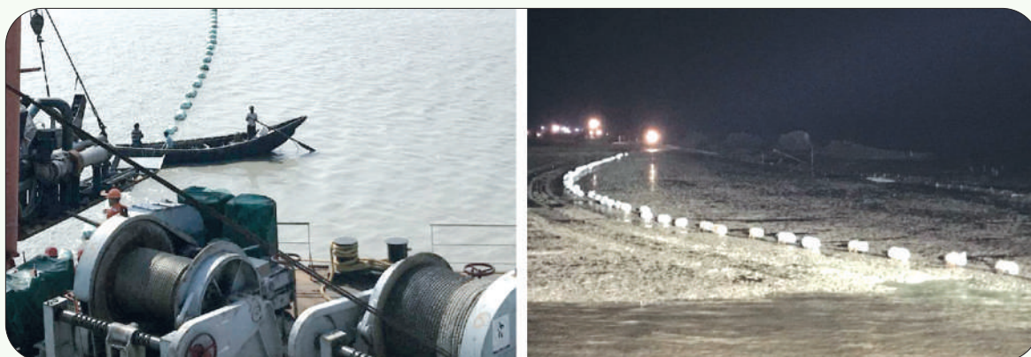
Laying of Submarine cable under the sea in order to connect Sandeep Island with national grid.
